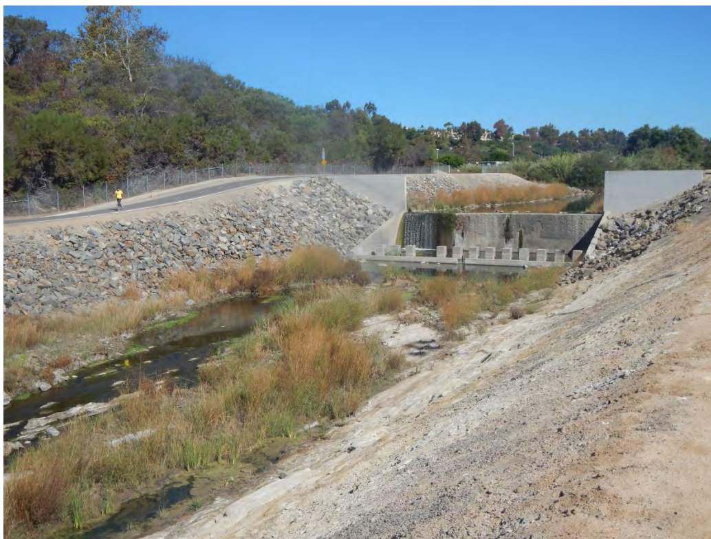
Photo 6 – Drop Structure to be Removed, Located U/S of Aliso Creek Road Bridge
