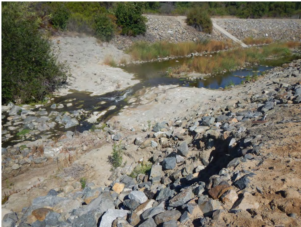
Photo 13 – Grouted Riprap Drop Structure to be Removed, Located D/S of Aliso Creek Road
