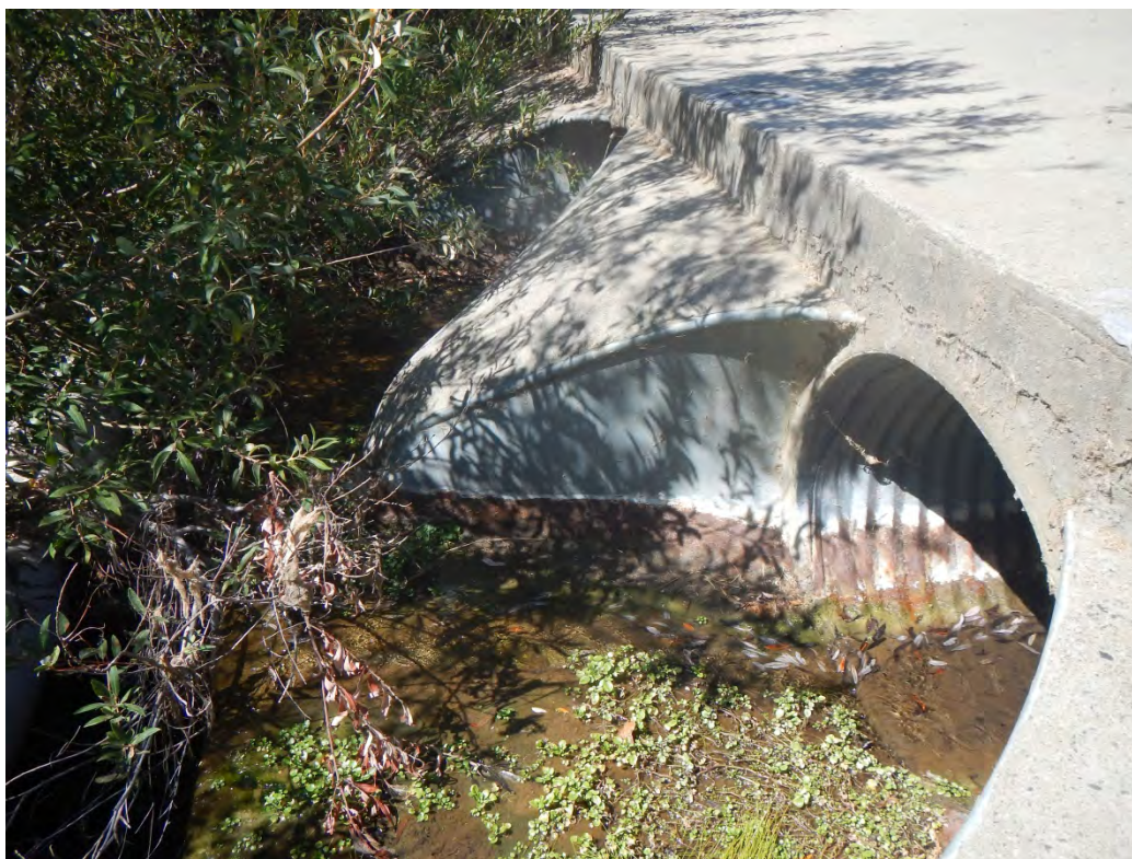
Photo 22 – D/S End of Wood Canyon Creek Culverts under Paved Trail at Aliso Creek Confluence ((3) 42”(W) x 30”(H) Elliptical CMPs)
