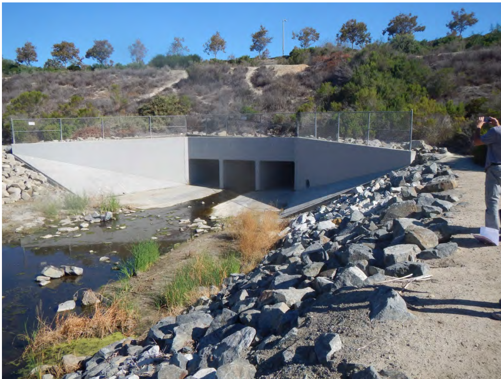
Photo 1 – D/S Face of RCB Culvert under Pacific Park Drive
