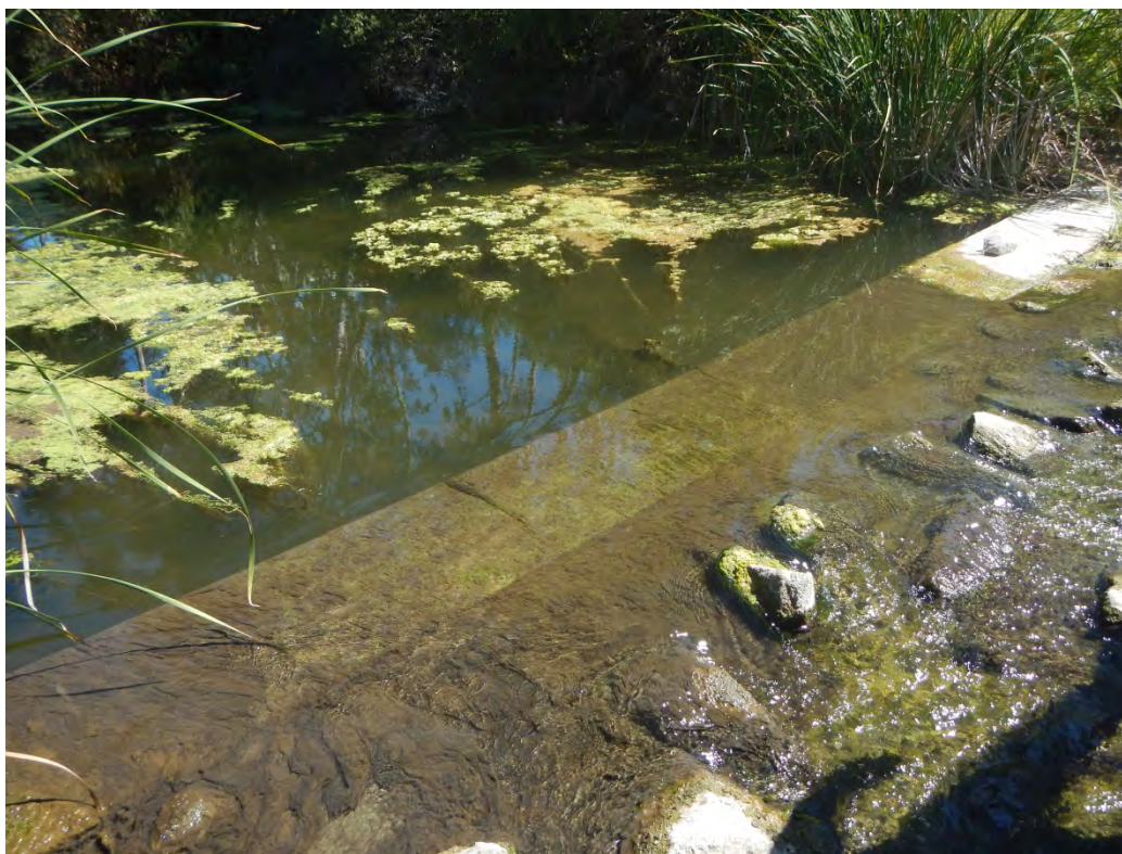
Photo 28 – U/S Limit of Grouted Riprap underneath SOCWA Coastal Treatment Plant Bridge
