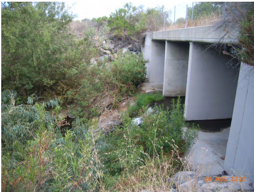
Photo 17 – Existing RCB Culvert along Sulphur Creek underneath Alicia Parkway
