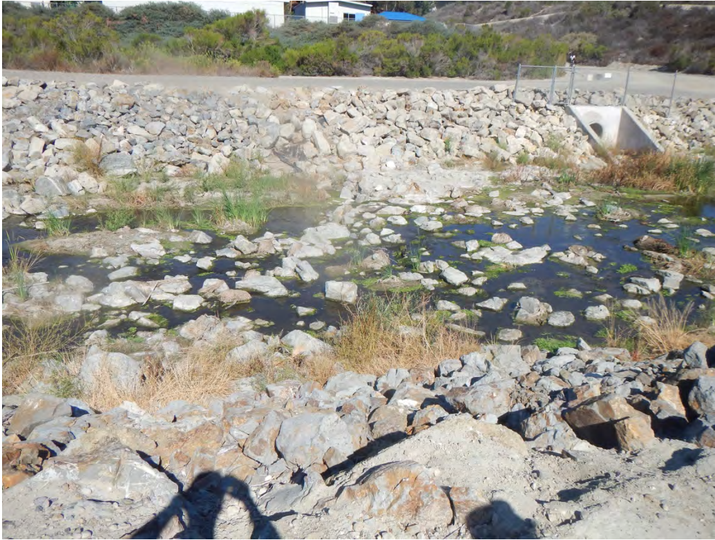
Photo 3 – Grouted Riprap across Streambed Possibly for Utility Crossing (approximately 180' D/S of Pacific Park Drive Culvert D/S Face)
