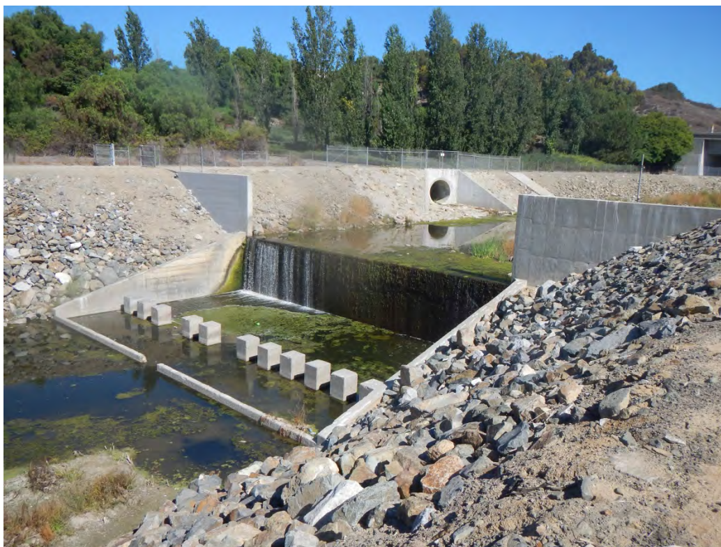
Photo 12 – Drop Structure to be Removed, Located D/S of Aliso Creek Road Bridge
