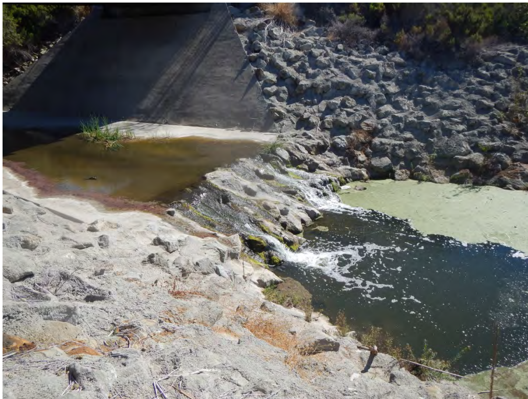
Photo 15 – Grouted Riprap Drop Structure Immediately D/S of AWMA Road Bridge
