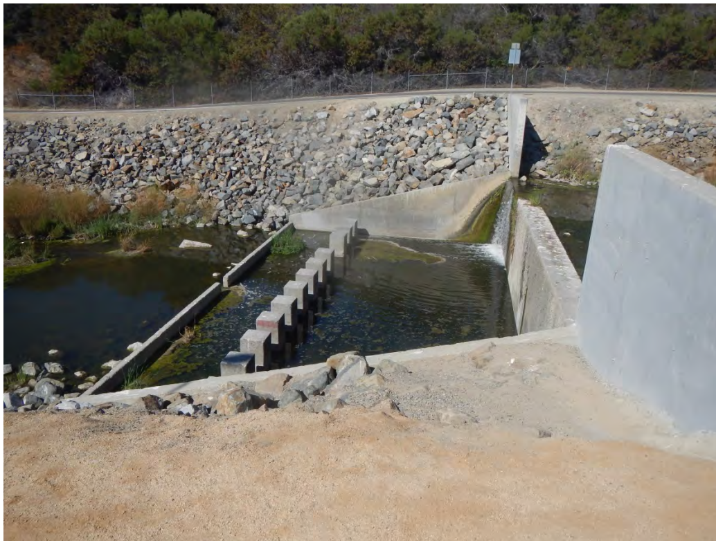
Photo 7 – Drop Structure to be Removed, Located U/S of Aliso Creek Road Bridge (Close-up)
