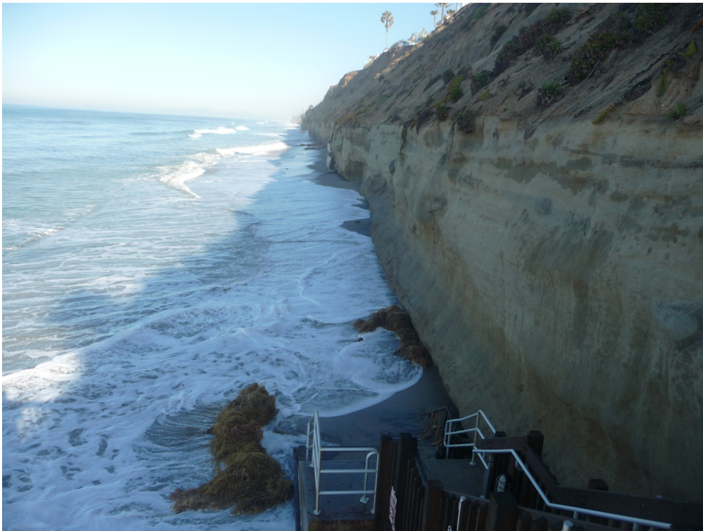
Figure 10.3-1 Wave Inundation at beach in Encinitas
