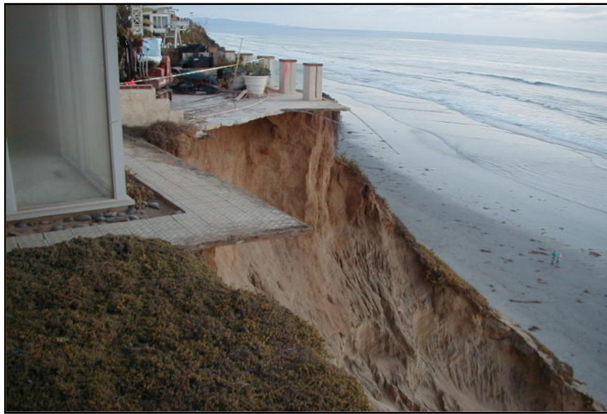
Figure 1.4-2 Example of damage to structure and land loss at bluff top edge
