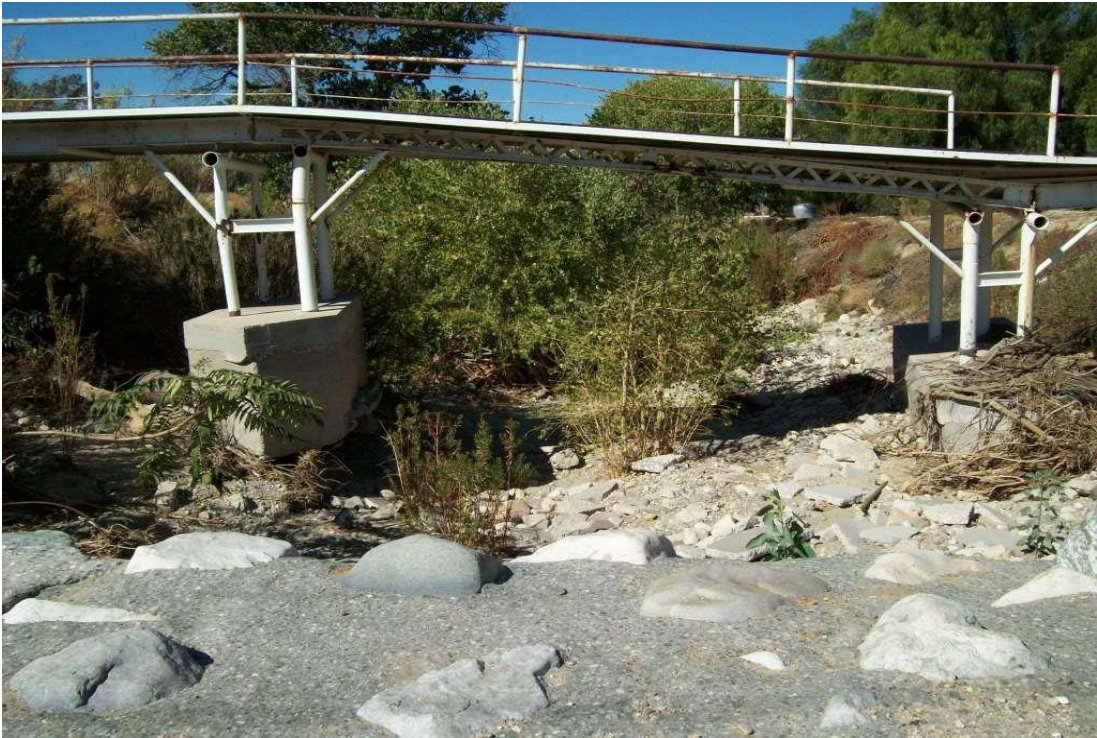
• Hacienda Road - Looking downstream from upstream side
