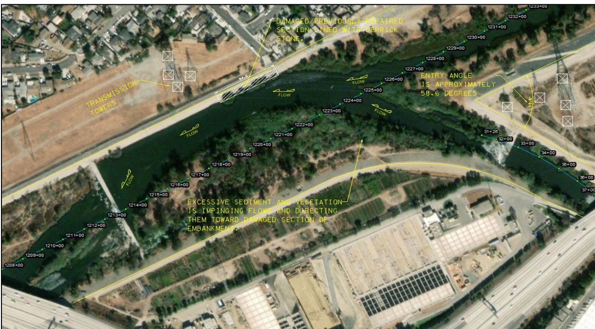
Figure 1.4-1 Excessive sediment and vegetation have directed flows at the levee's embankment increasing risk of failure.
