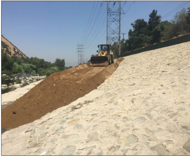
Figure 2.1-3 Example of temporary access ramp
