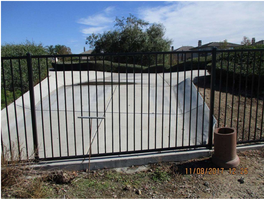
Fig. 38.—Spillway outlet of small detention basin 100 ft north of the River Road Dike conceptual alignment. 8 November 2017.
