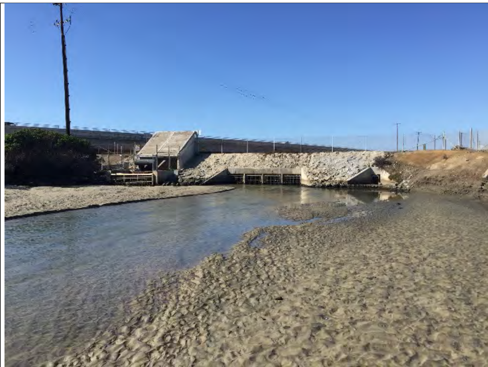
Santa Ana River Tide Gate
