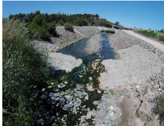
Photo 2.3-2 At the upstream end of the Proposed Project Area, Aliso Creek has a soft bottom and engineered-compacted fill banks and armored side slopes.
