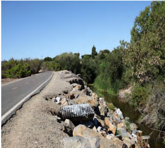
Photo 2.17-1 Culverts as outfalls deliver local runoff to the Creek
