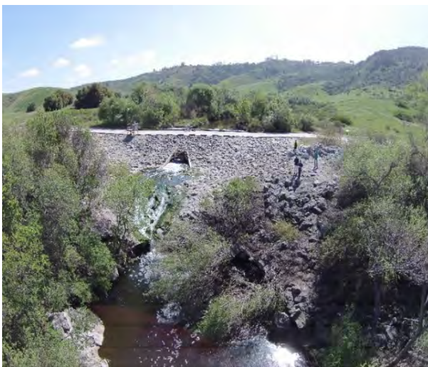
Photo 2.1-4 The ACHWEP is a grade control and overflow structure in the Wilderness Park designed to slow water upstream of the structure.
