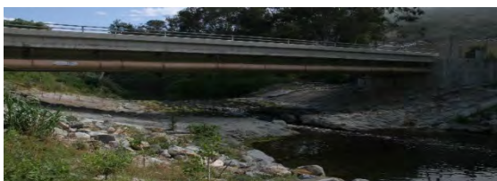
Photo 2.17-4 Bridges are also conduits for water and waste water pipelines.
