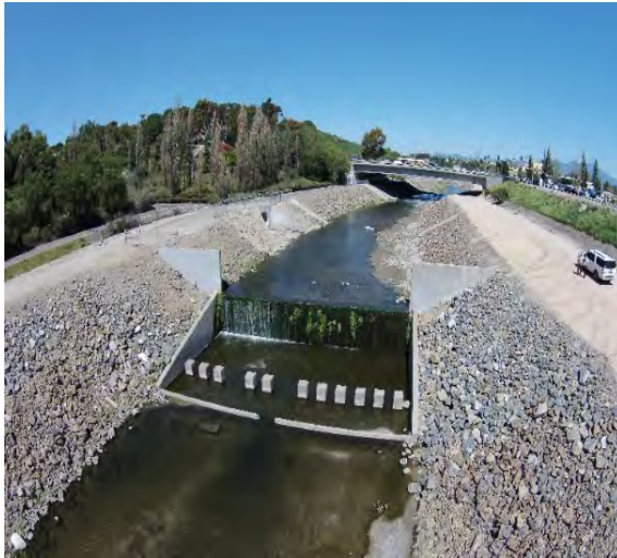
Photo 2.3-3 Several drop structures along Aliso Creek within the Proposed Project area were established for flood control purposes.
