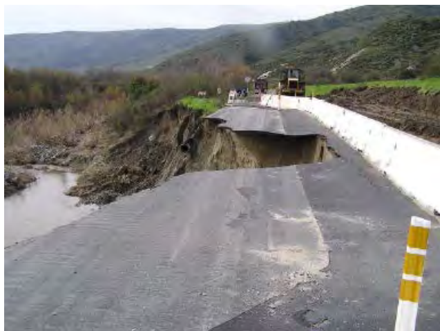
Photo 5.2-1 Continued erosion and downcutting of side slopes along the west side of the creek. Bank erosion has caused the road to be moved further west towards the canyon hillsides.
