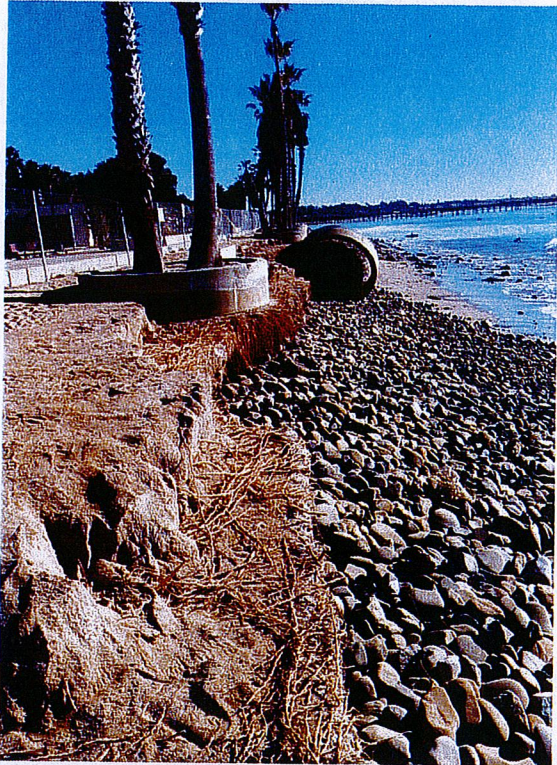
December 2015 (Pre Discharge): Looking east from approximately Station 2+70.
