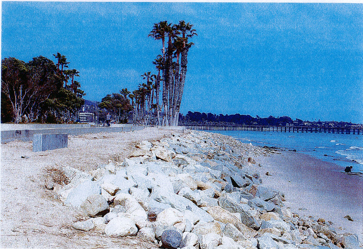
March 2016 (Post Discharge): Looking east from approximately Station 3+00.
