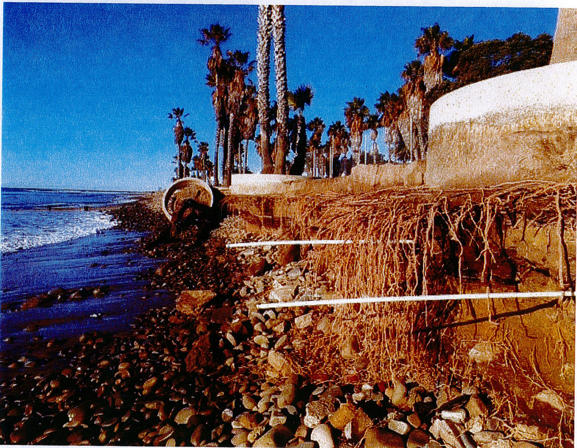
December 2015 (Pre Discharge): Looking west from approximately Station 4+60.
