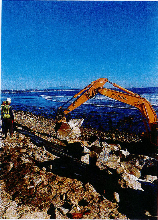
1.5 to 3 ton rock being placed along the center portion of the project limits by excavator. (2016)
