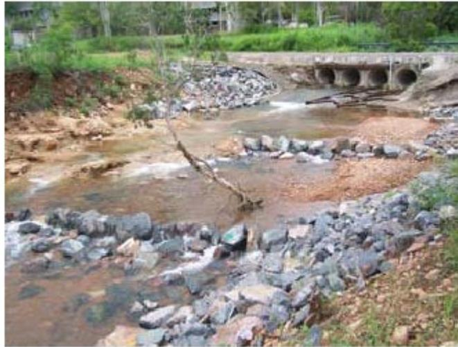
**Figure 3.6A – Typical Series of Transverse Ridge Rock in Creek (Kapitzke 2010)**
