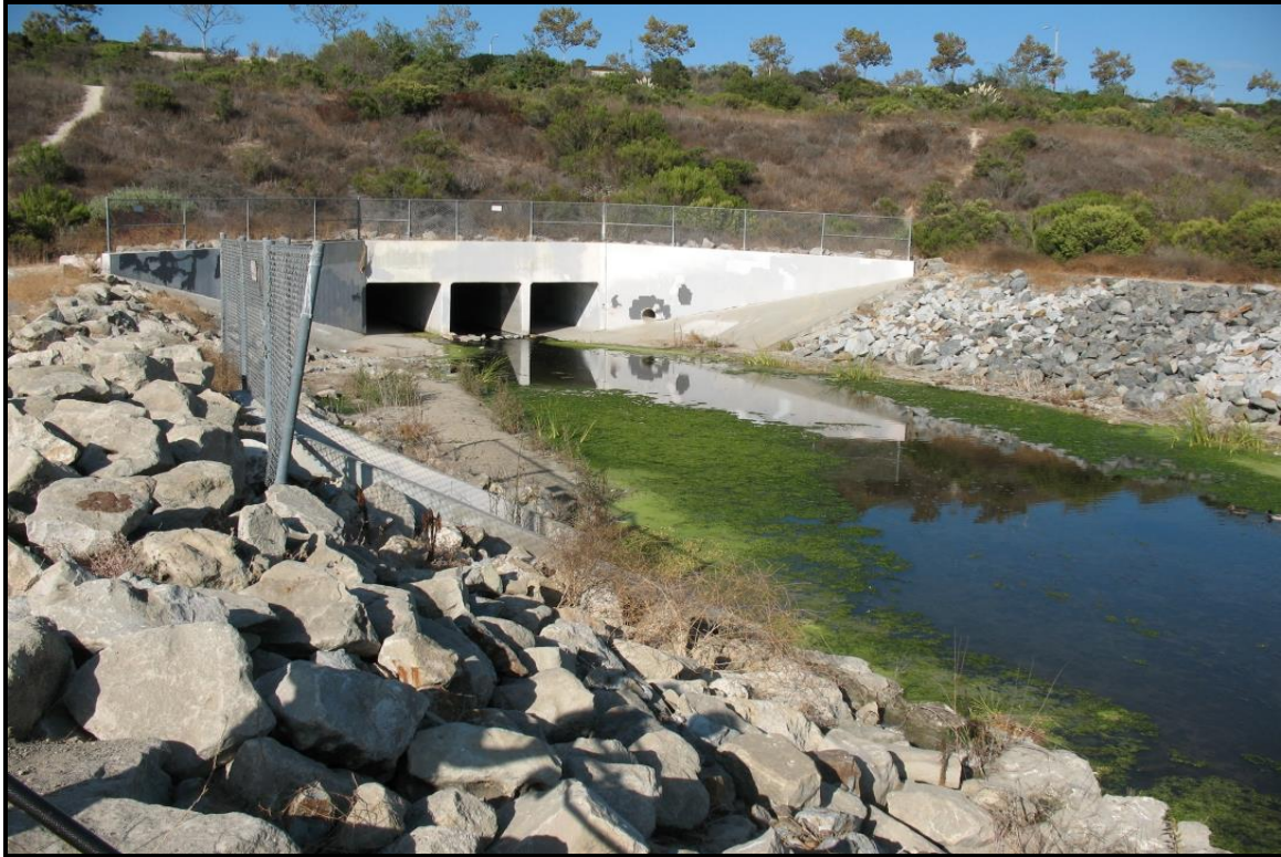
Figure 3-62. Upstream view of three 8-ft x 8-ft concrete box culverts under Pacific Park Drive
