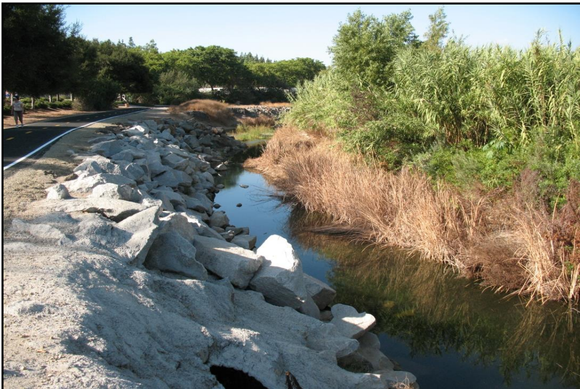
Figure 3-63. Riprap bank protection and bank scalloping between riprap protection
