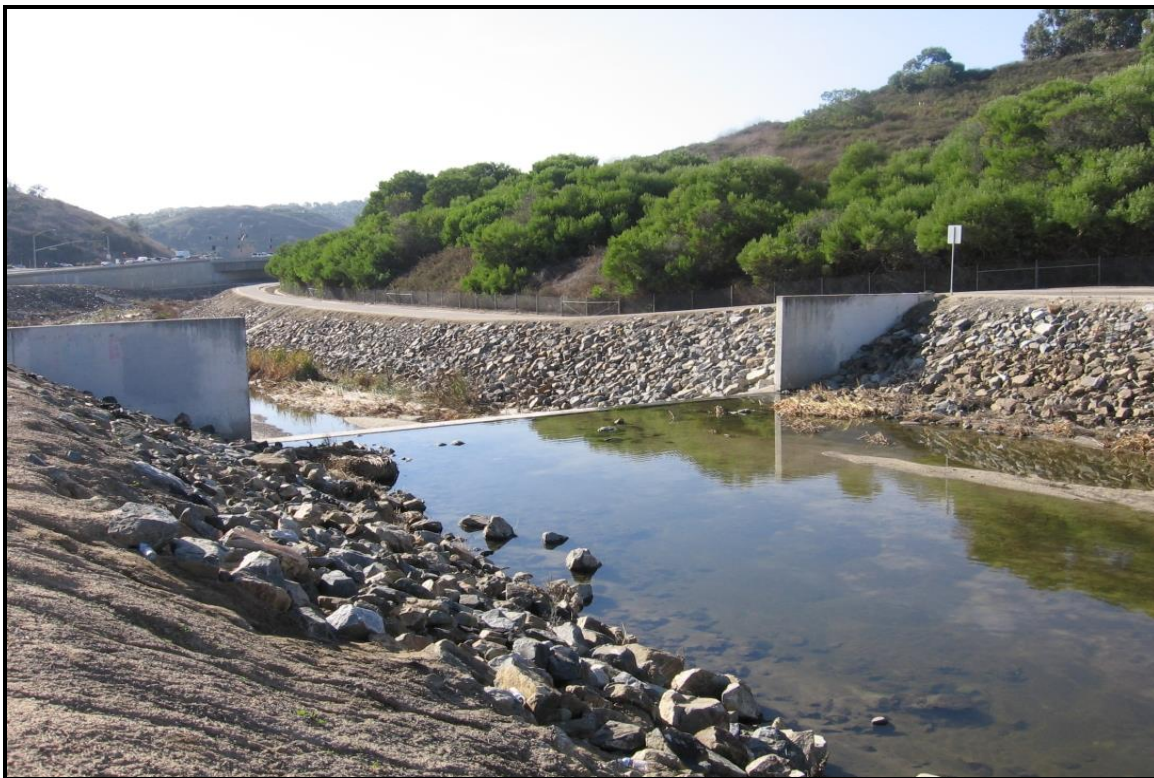
Figure 3-56. Engineered channel and riprap-protected banks typical of Reach 10
