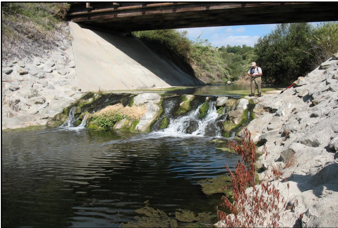
Figure 3-53. A WMA Road grade control at upstream end of Reach 9
