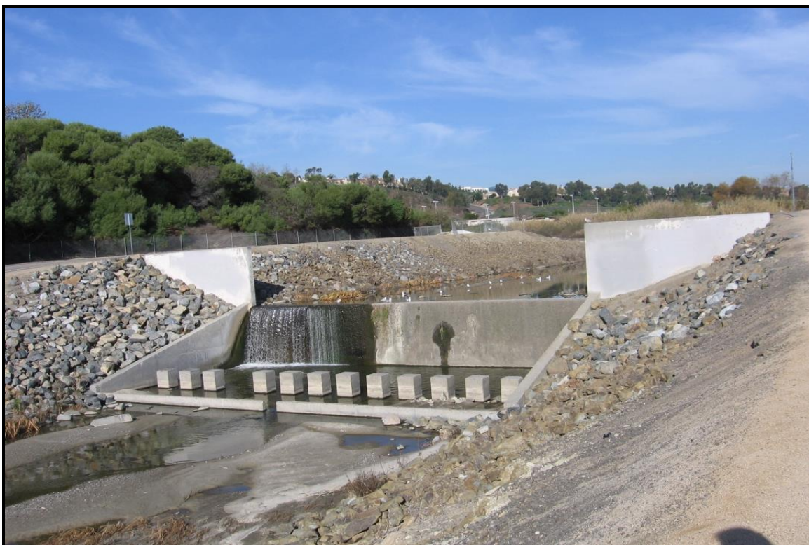
Figure 3-55. Concrete drop structure in Reach 10 (drop is 10 feet)
