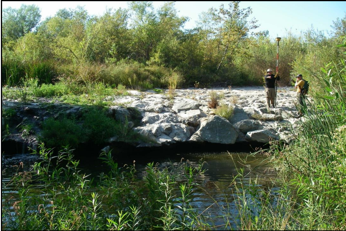
Figure 3-57. Grouted riprap grade control at crossing of water supply pipelines
