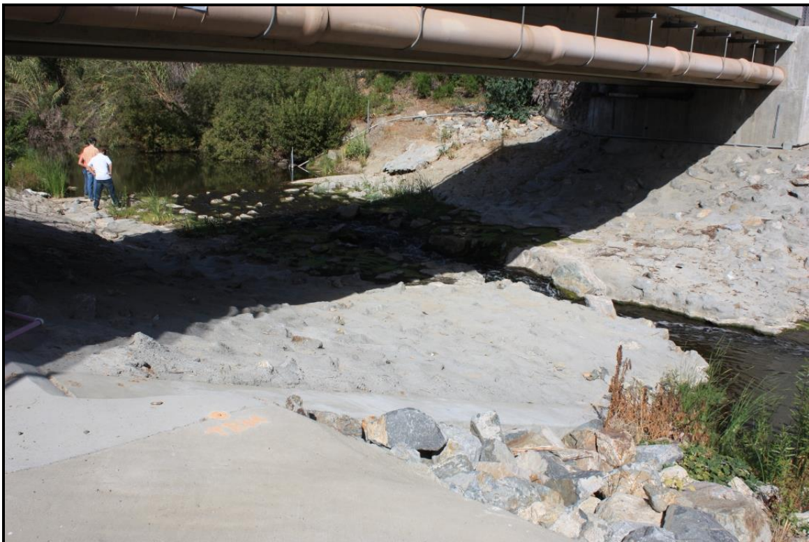
Figure 3-29. SOCWA bridge grade control and concrete sill
