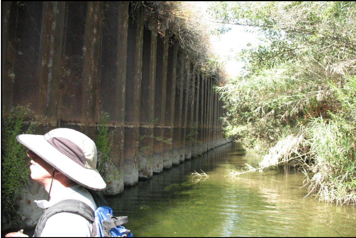
Figure 3-59. Upstream view of sheet pile wall along the right bank
