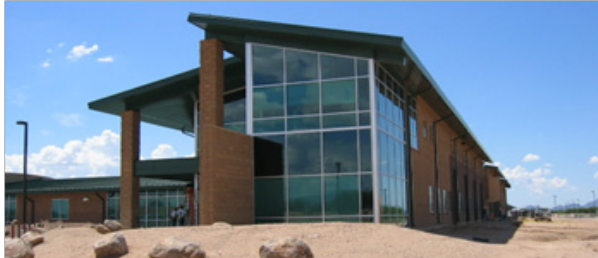
Tucson Sector Headquarters Admin Bldg
