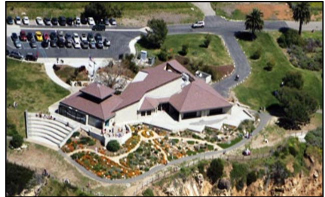
Figure 1 shows an aerial photo of the Point Vicente Interpretive Center. (Source: www.SanPedro.com)
