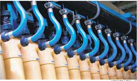
Water is pumped through microfiltration membrane filtration modules at the Advanced Water Purification Facility in University City.
