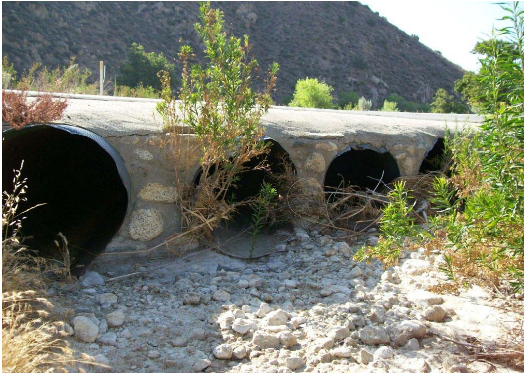
• Aliso Canyon Road – Looking downstream at upstream side
