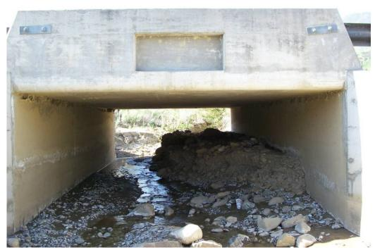
• Sycamore – Downstream side of culvert showing sediment blocking ¼ of conveyance area
