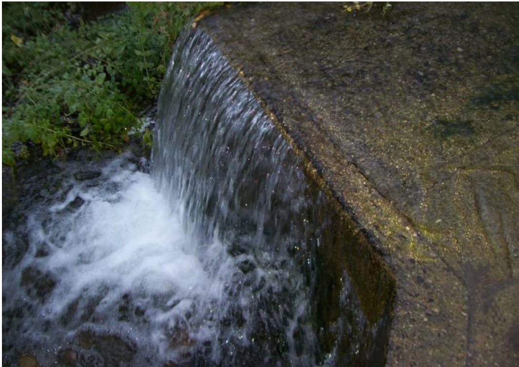
• Bouquet Cyn Rd 2 – Looking upstream from downstream side buried culvert
