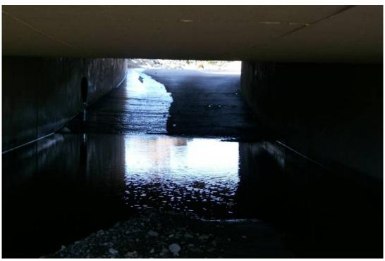
North Bank and Elba – Downstream side of culvert looking upstream – shows slope break under road
