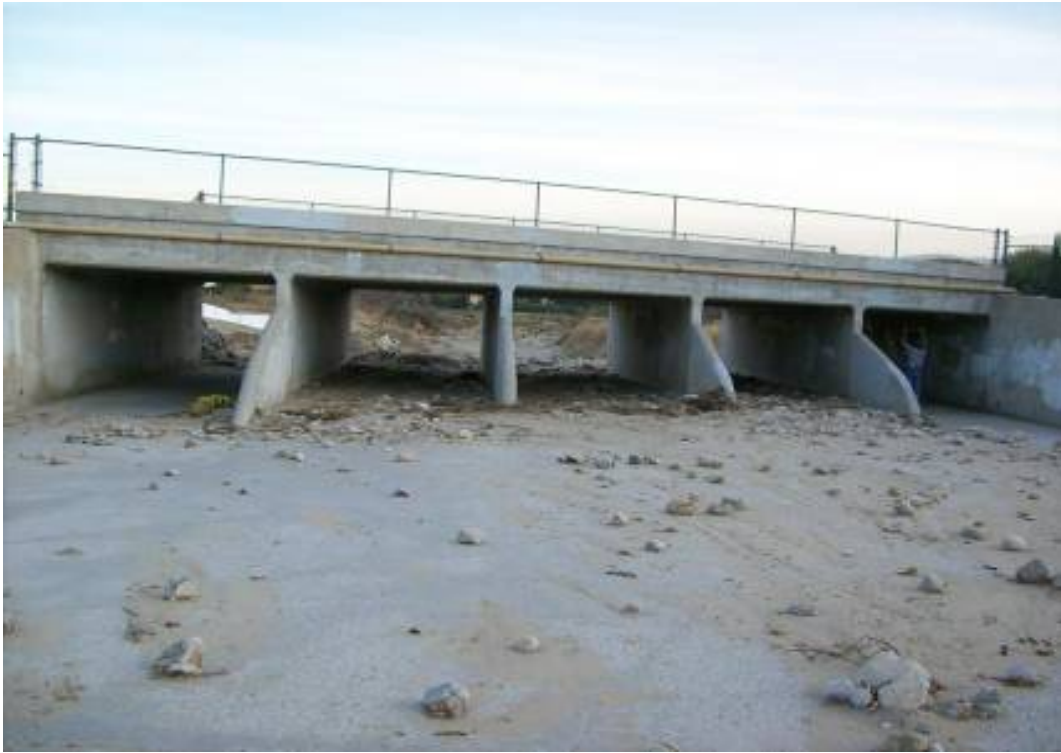
• Romero Road - Looking downstream from upstream side
