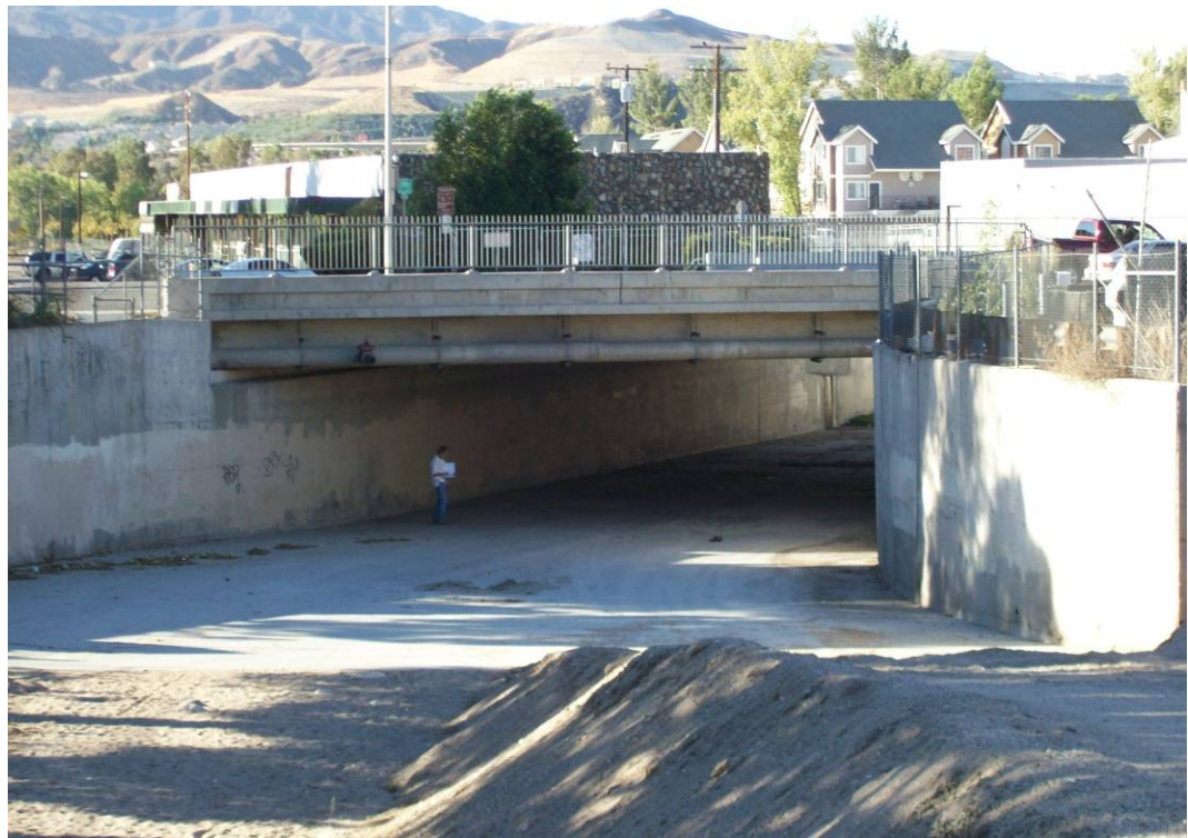
• Soledad Canyon Rd – Looking downstream from upstream side
