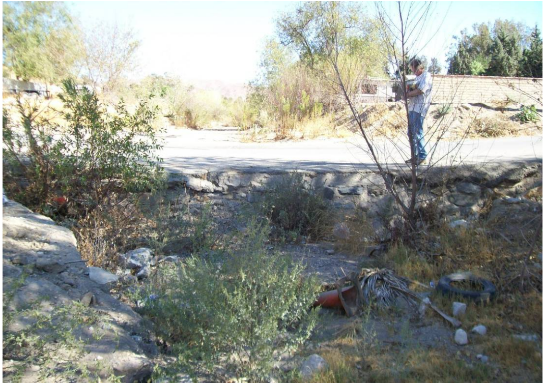
• Arline St – Looking upstream from downstream side
