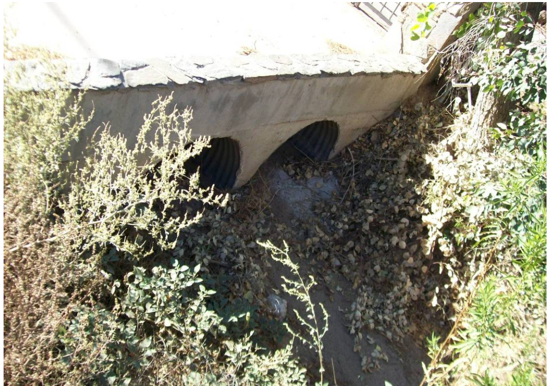
• Private Driveway 5— Looking downstream from upstream side
