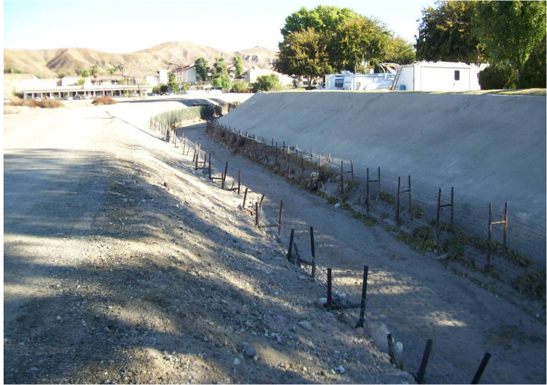
• Soledad Canyon Rd – Looking upstream
