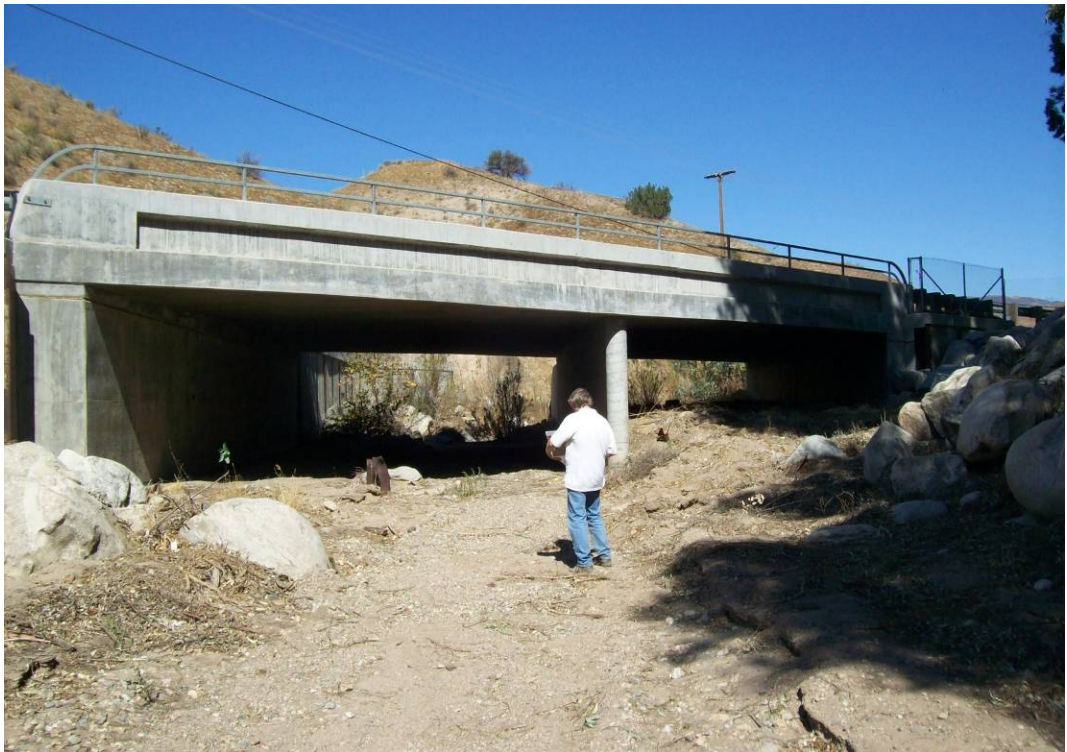
• Sierra Hwy 3 – Looking upstream from downstream side
