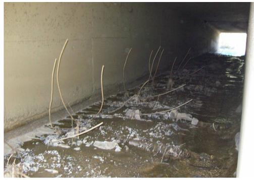
• Highway 126 – Downstream side of culvert looking at west barrel exposed rebar
