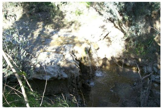
• Highway 126 – Drop (scour hole) downstream of bridge
