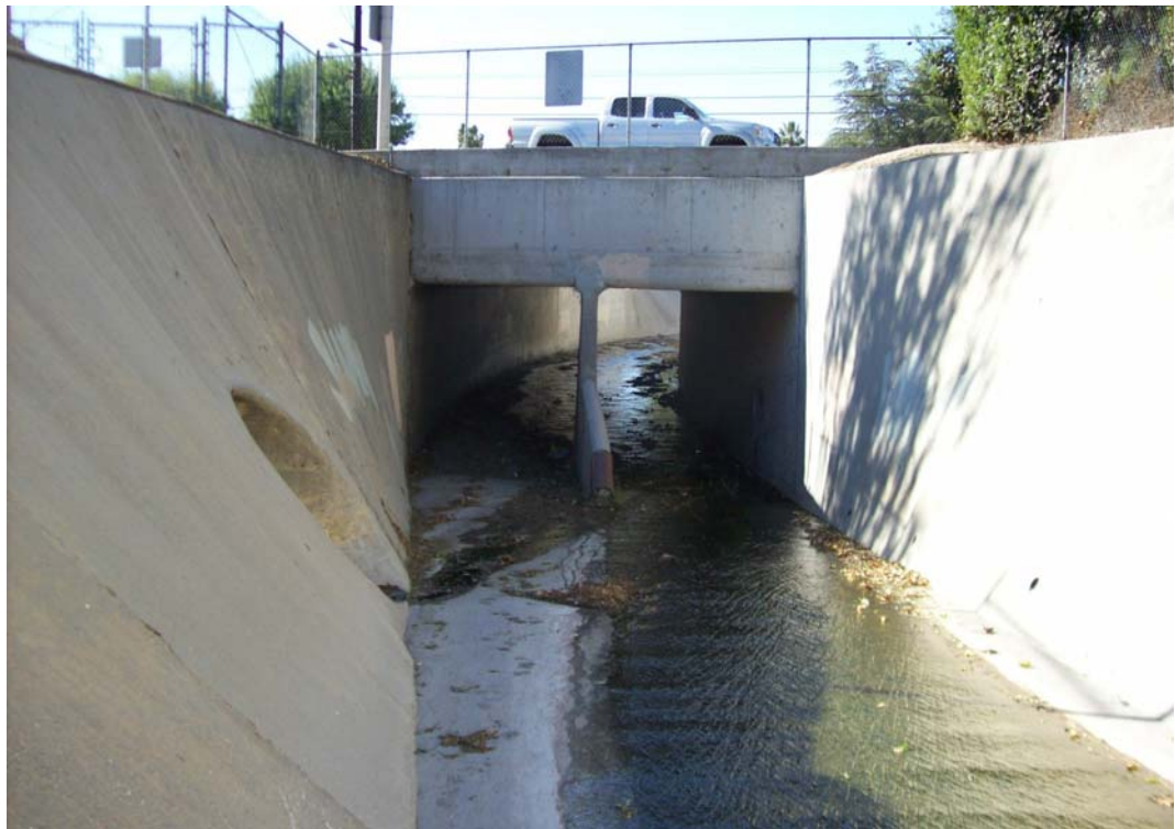
• Bouquet Cyn Rd – Looking downstream from upstream side
