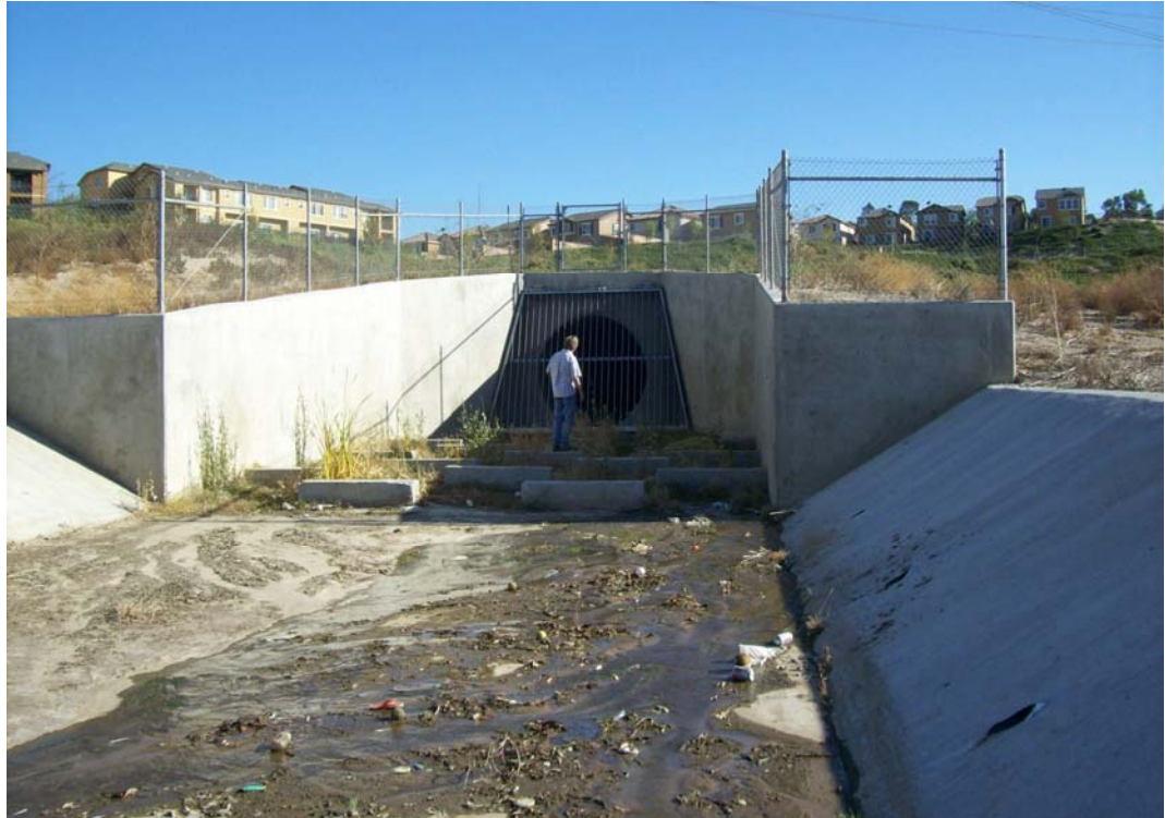
• Debris Basin – Looking upstream
