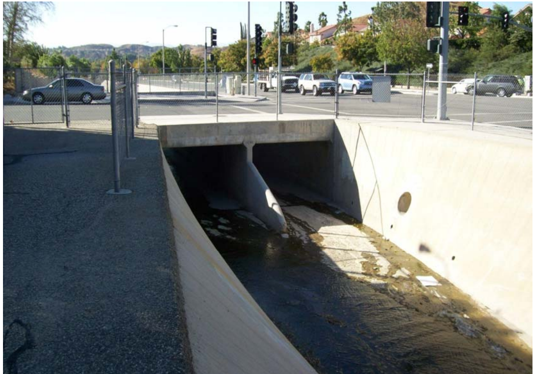
• Rodgers Rd – Looking downstream from upstream side
