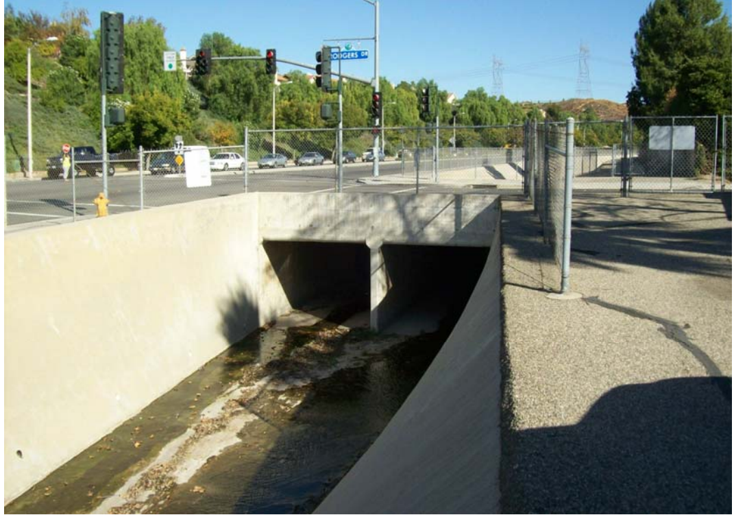
• Rodgers Rd – Looking upstream from downstream side
