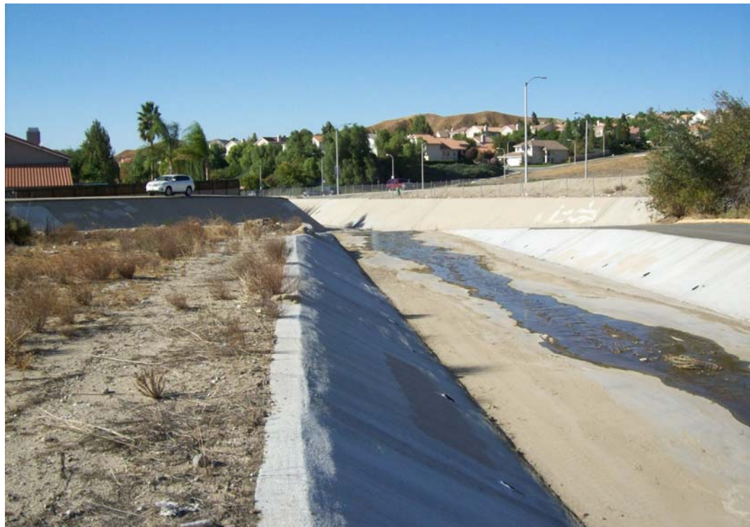
• Debris Basin – Looking downstream
