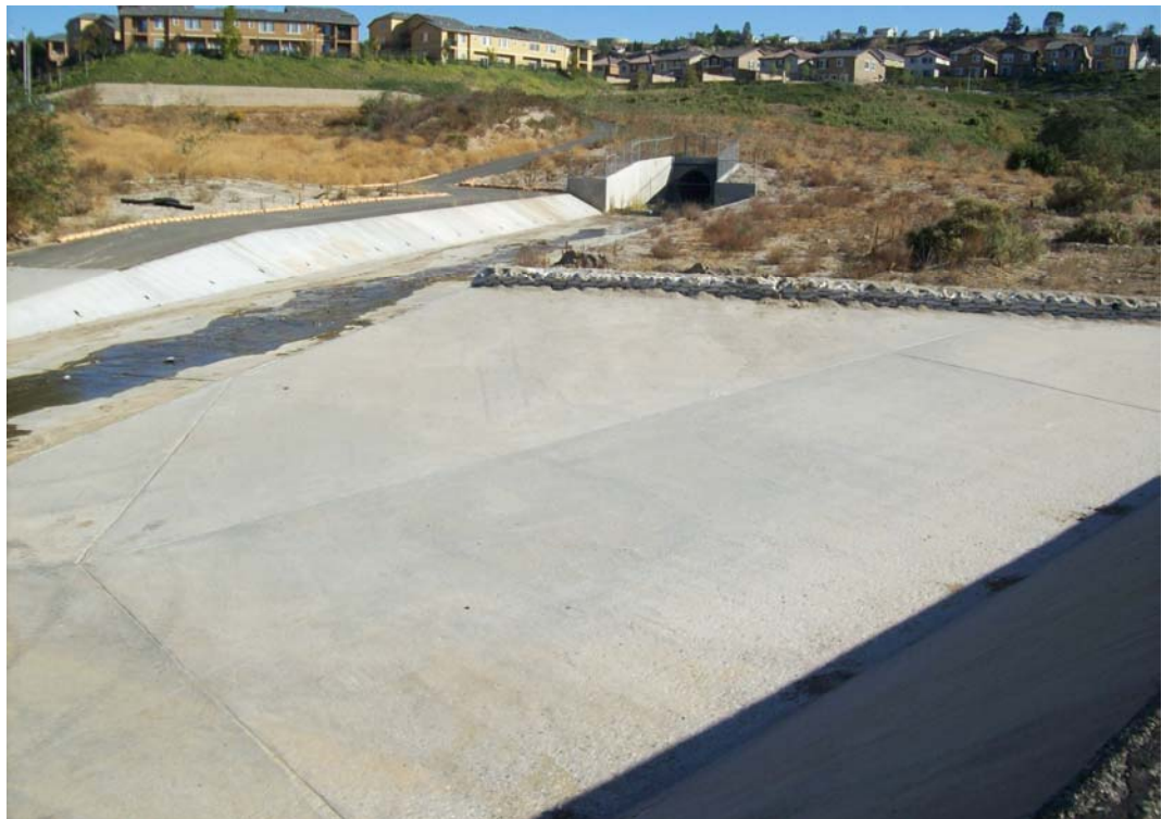
• Debris Basin – Looking upstream
