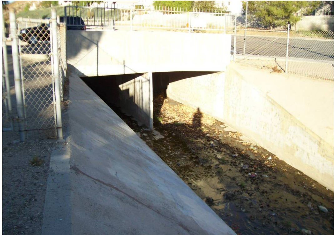
• Grandifloras Rd – Looking upstream from downstream side
