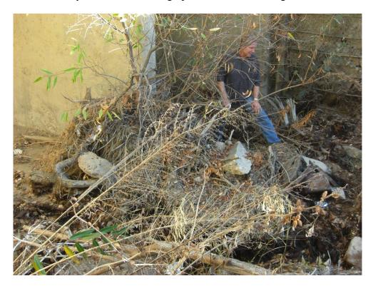
Wheeler Canyon Rd\_B – Upstream face of the bridge (debris pile upstream of pier)
