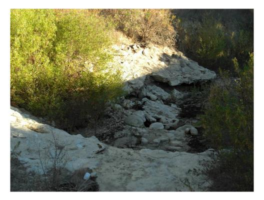
Wheeler Canyon Rd\_B – Looking downstream from the bridge (concrete channel bed collapsed)
