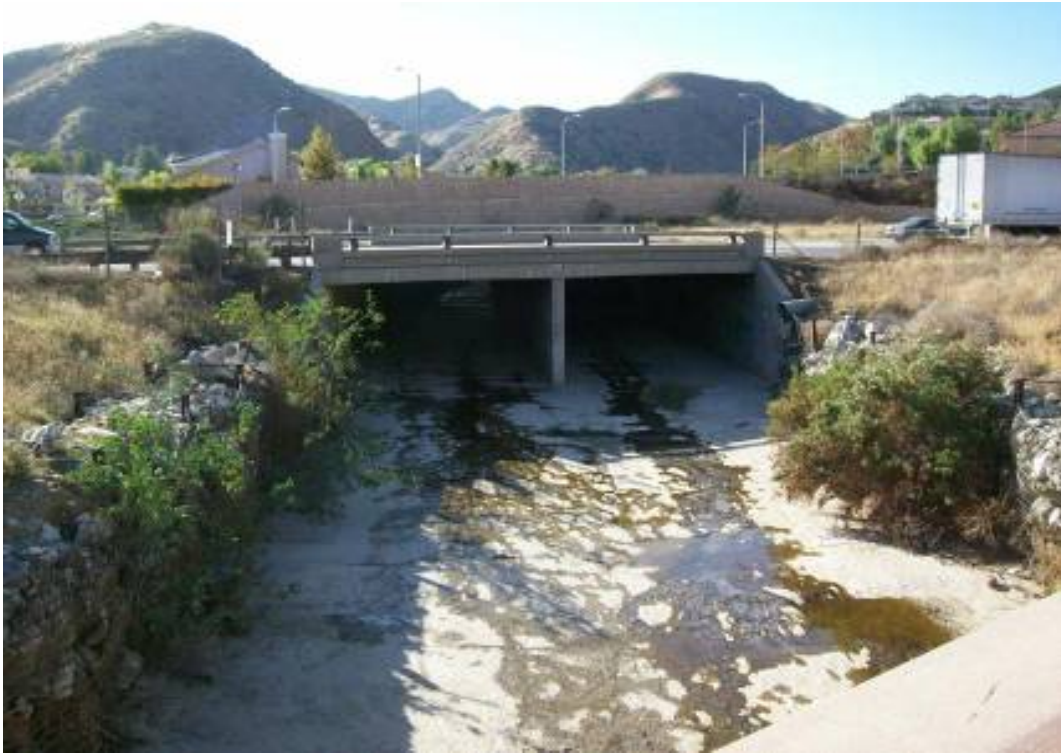
• Interstate 5 - Looking upstream from downstream side of bridge
