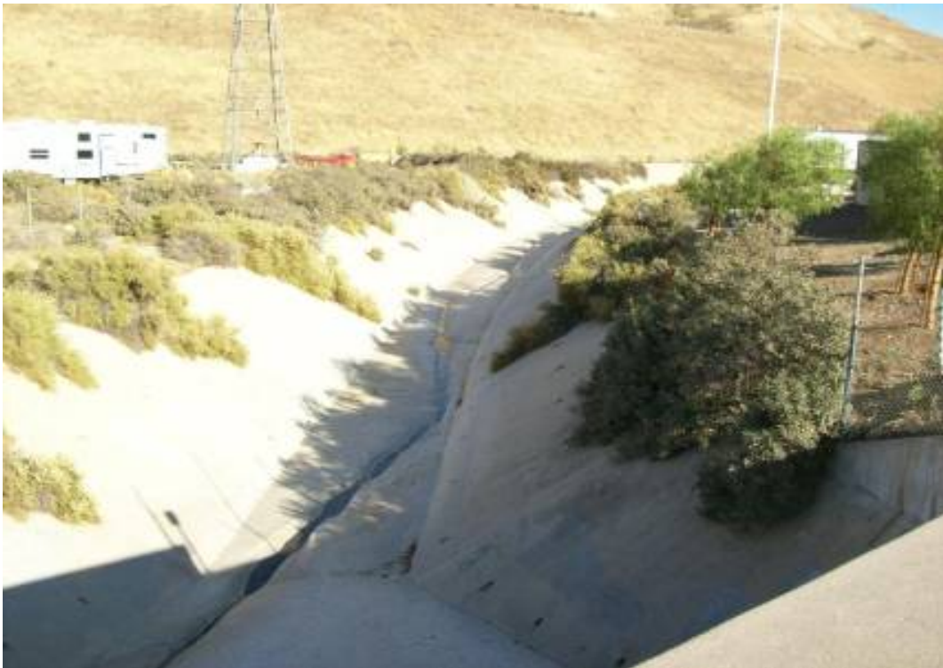
• Castaic Road - Looking downstream
