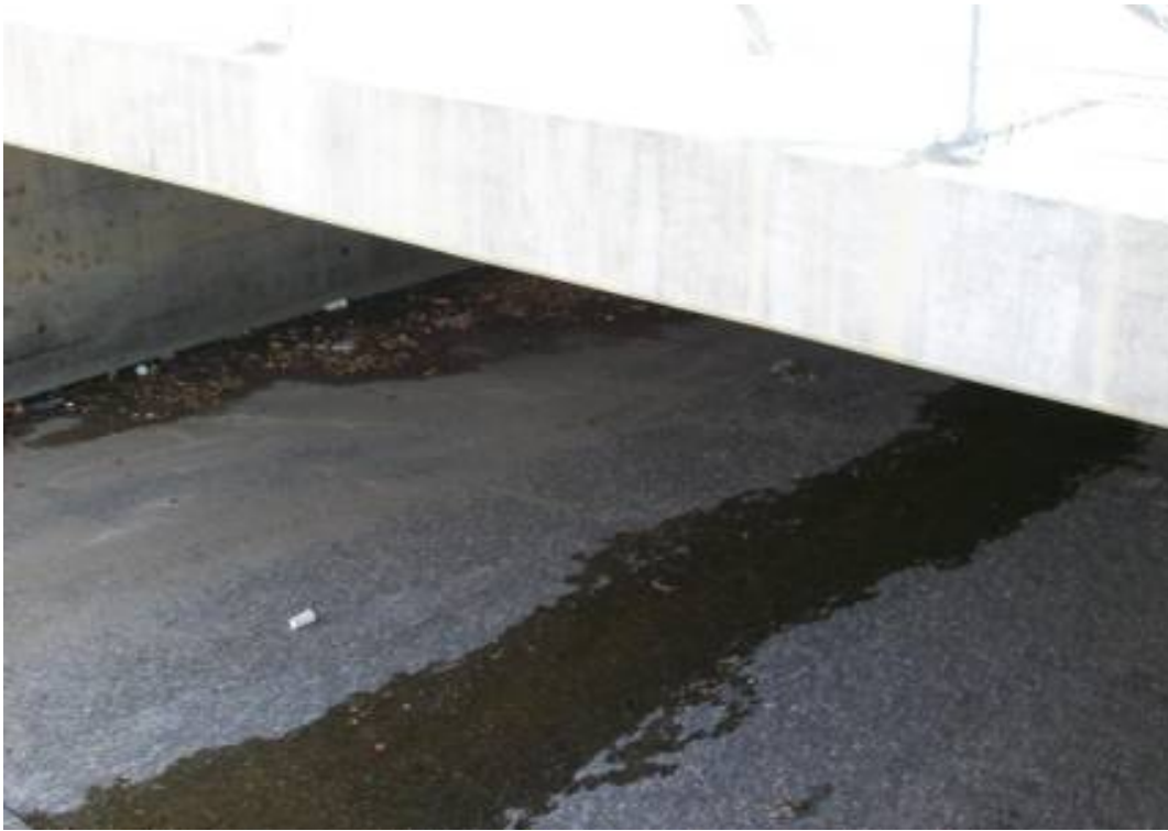
• Ridge Route – Looking at upstream side
