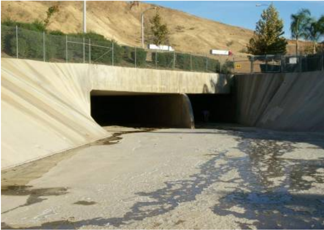
• Old Road - Looking downstream from upstream side
