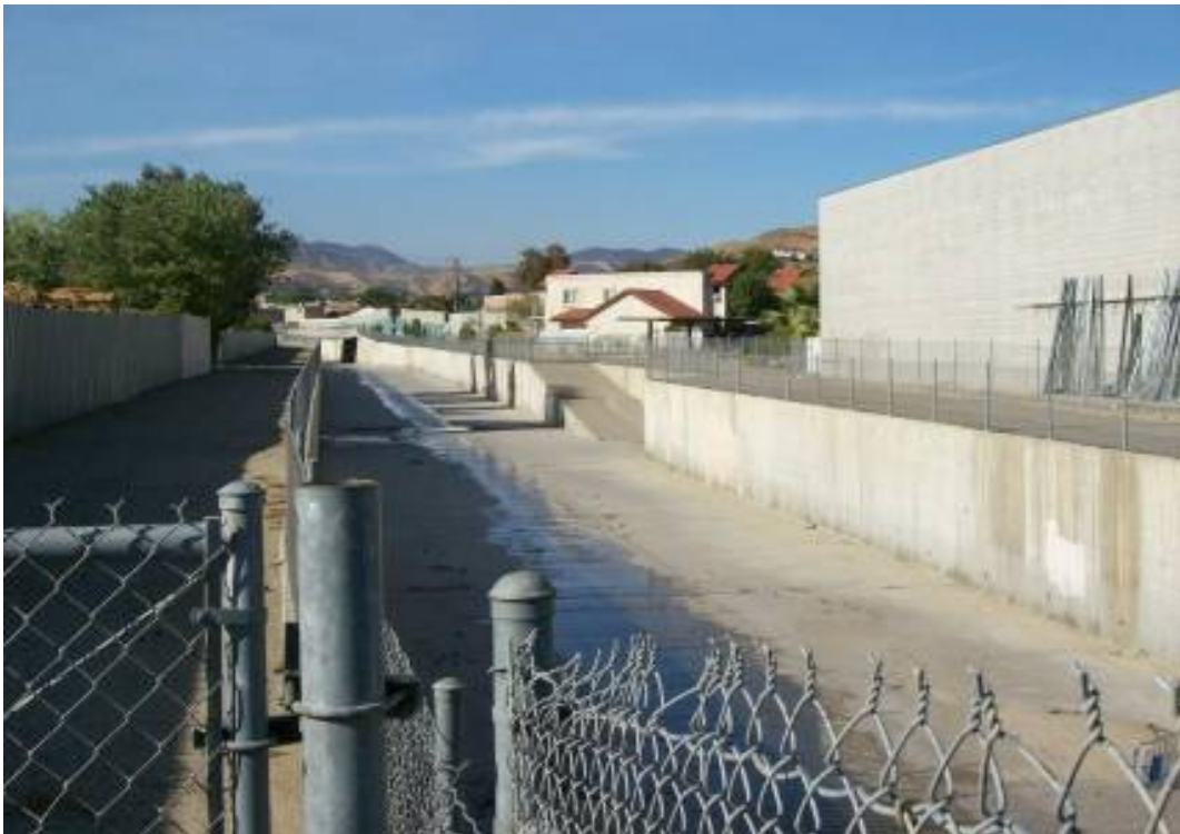
• Ridge Route - Looking upstream
