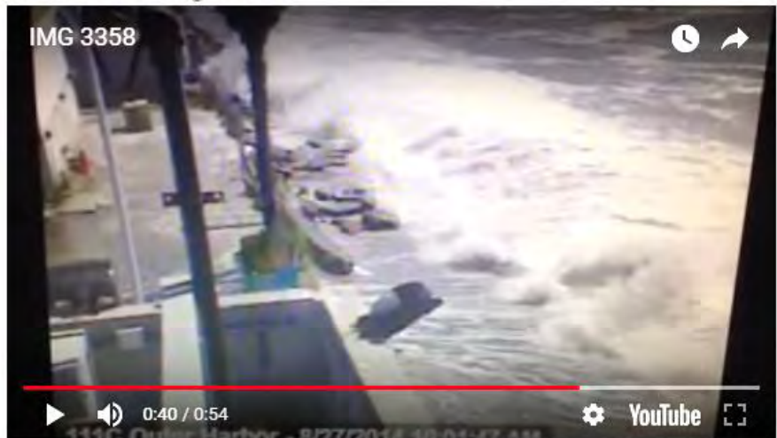
South Swell Damage 8-27-14
