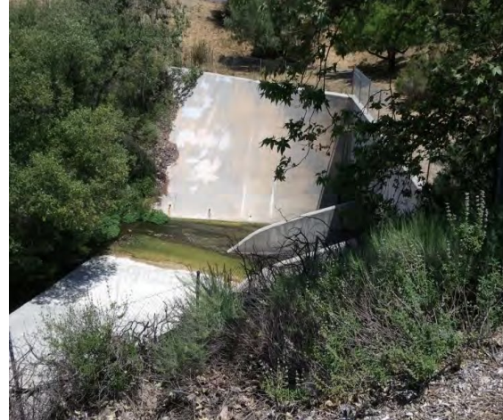
View upstream from Lost Hills Rd. showing wing walls.
