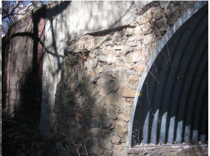
0037. South culvert abutment, mortared rock, measure, wood retaining wall, facing northwest. 02/26/2013
