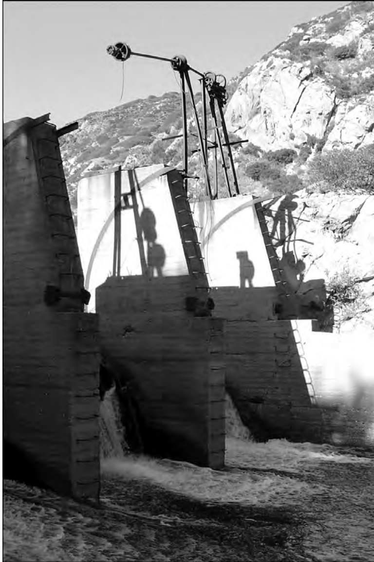
Figure 14. Buttresses 3, 4, and 5 and the spillway apron.
