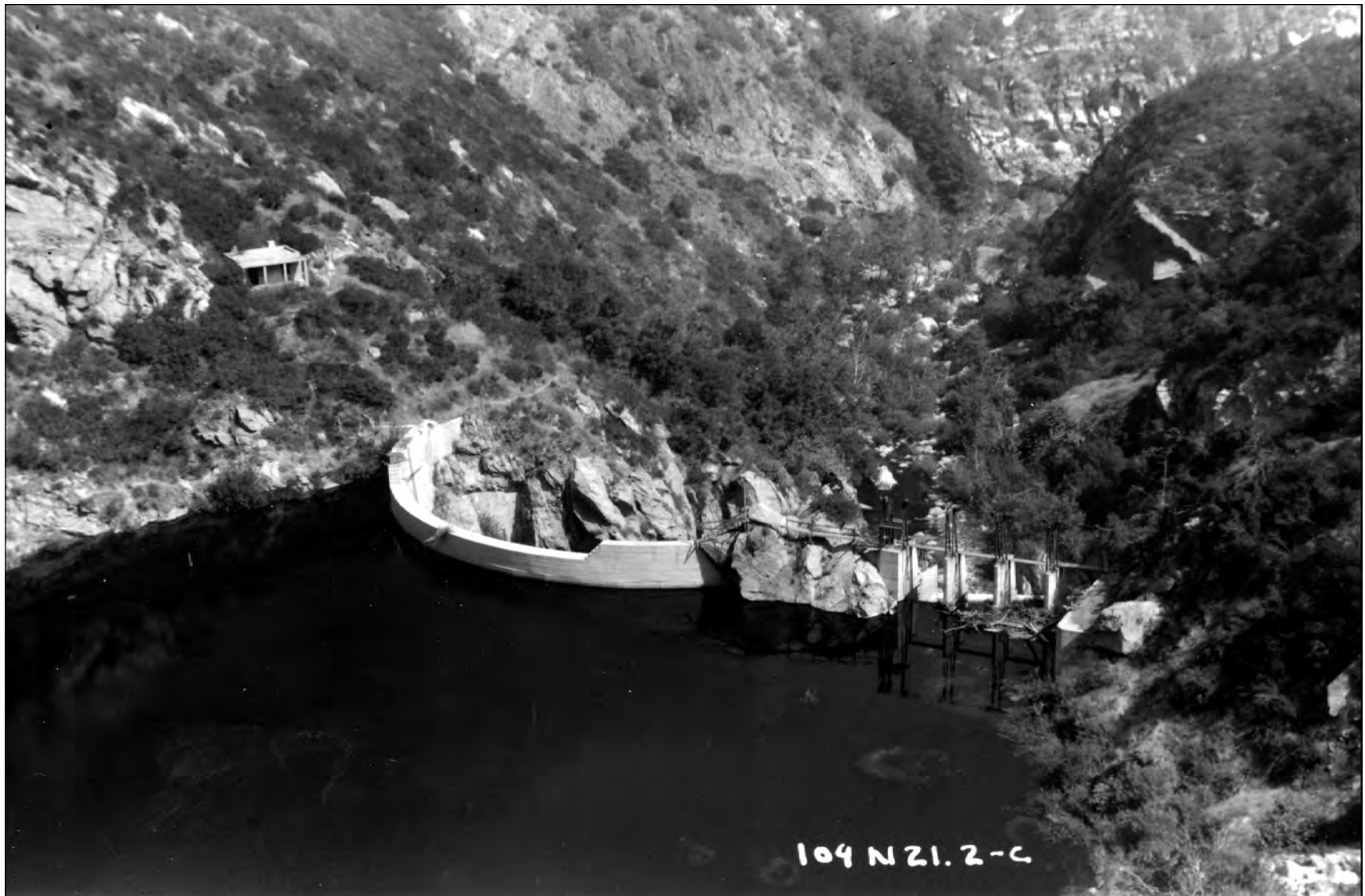
Figure 6. View of the dam to the south, October 3, 1952. The center section of the dam is 5 feet lower than the stepped ends. The dam keeper's house can be seen above the northern end of the dam (Los Angeles County Flood Control Department photograph, courtesy of Ronald L. Rindge).
