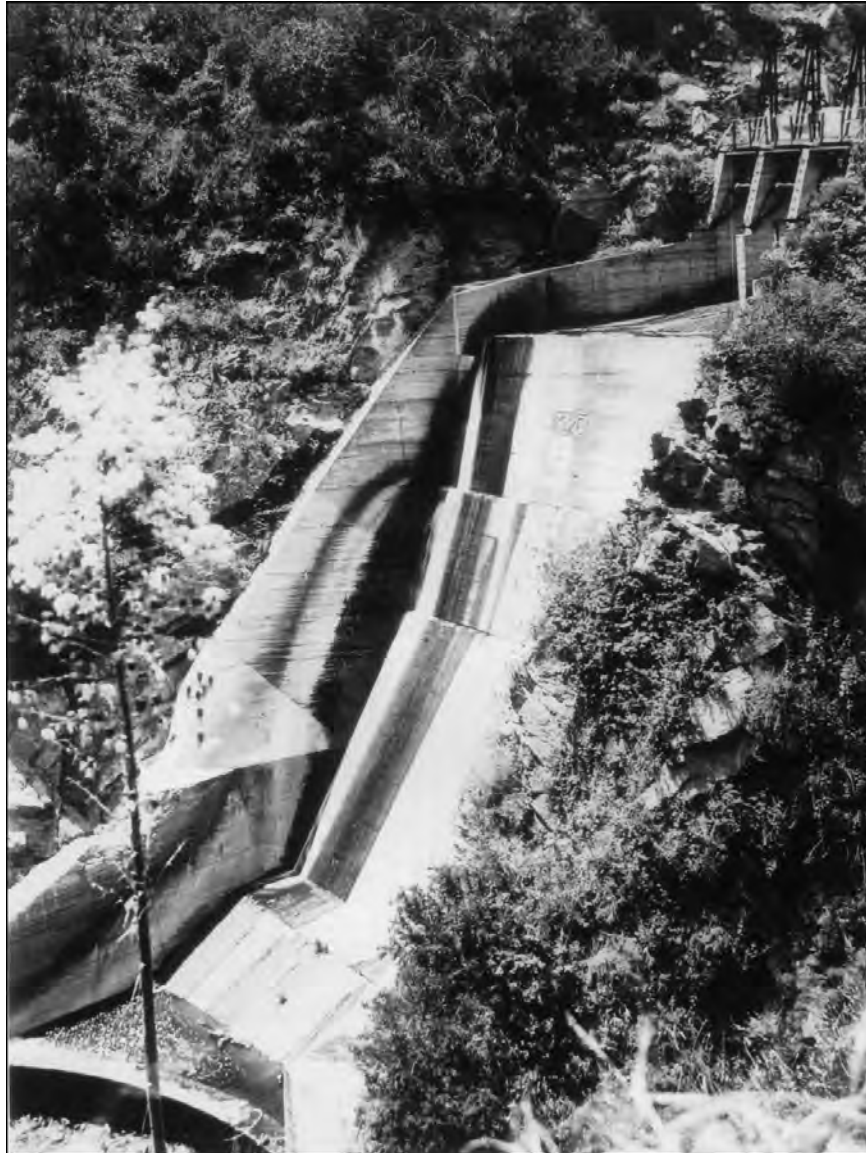
Figure 10. The angled levels of the spillway are evident from this photograph, taken ca. 1926 (Malibu Water Company photograph, courtesy of Louis T. Busch).
