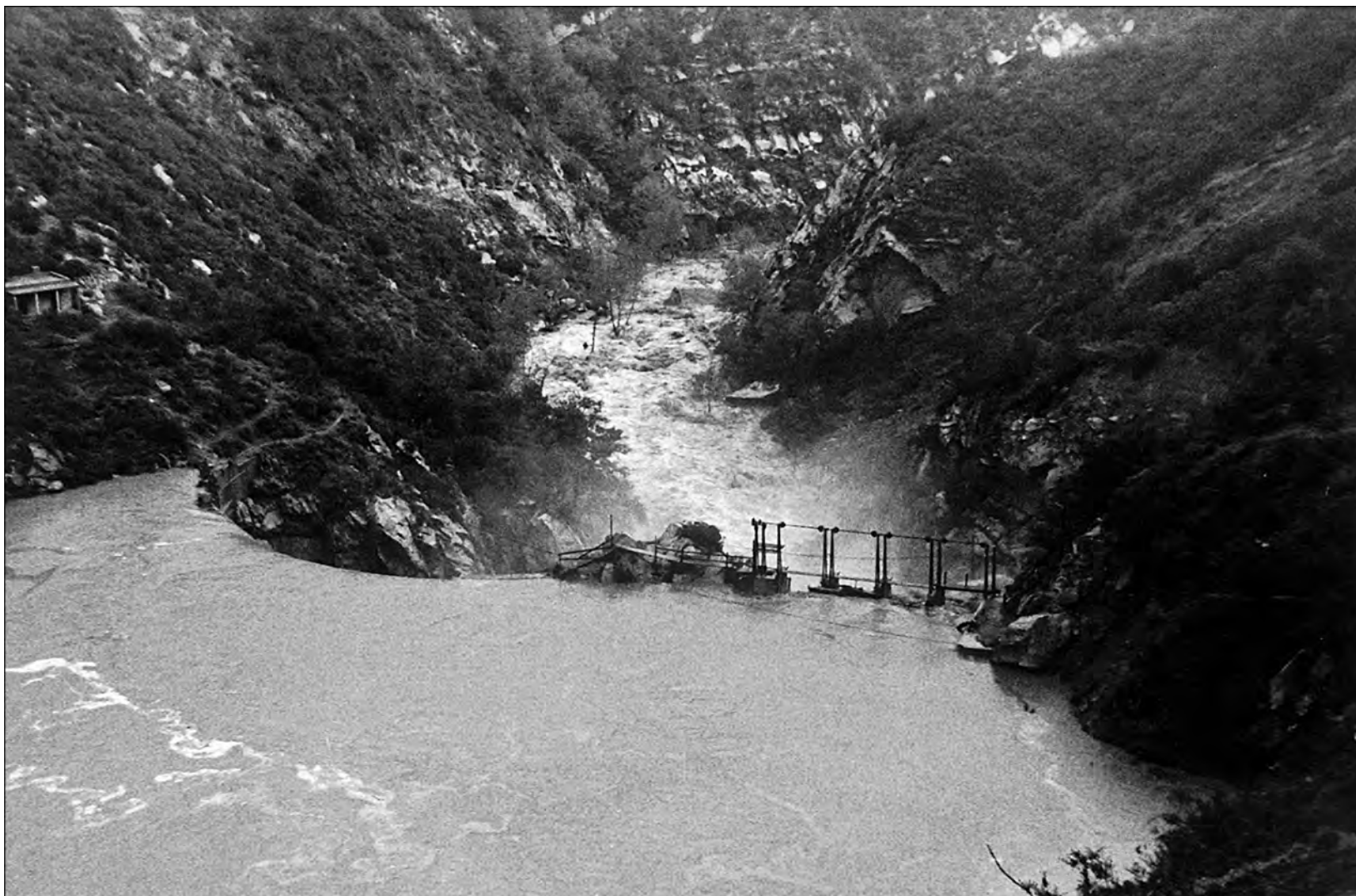
Figure 9. East view shows the spillway and the wooden access walkway. The dam keeper's house is clearly visible on the north side above the dam. Thought to have been taken sometime in the 1930s or 1940s, this photograph shows the creek in flood stage, with water up to the 5-foot level above the dam's lip (photograph courtesy of Malibu Lagoon Museum/Historic Adamson House, No. MD:83-7).
