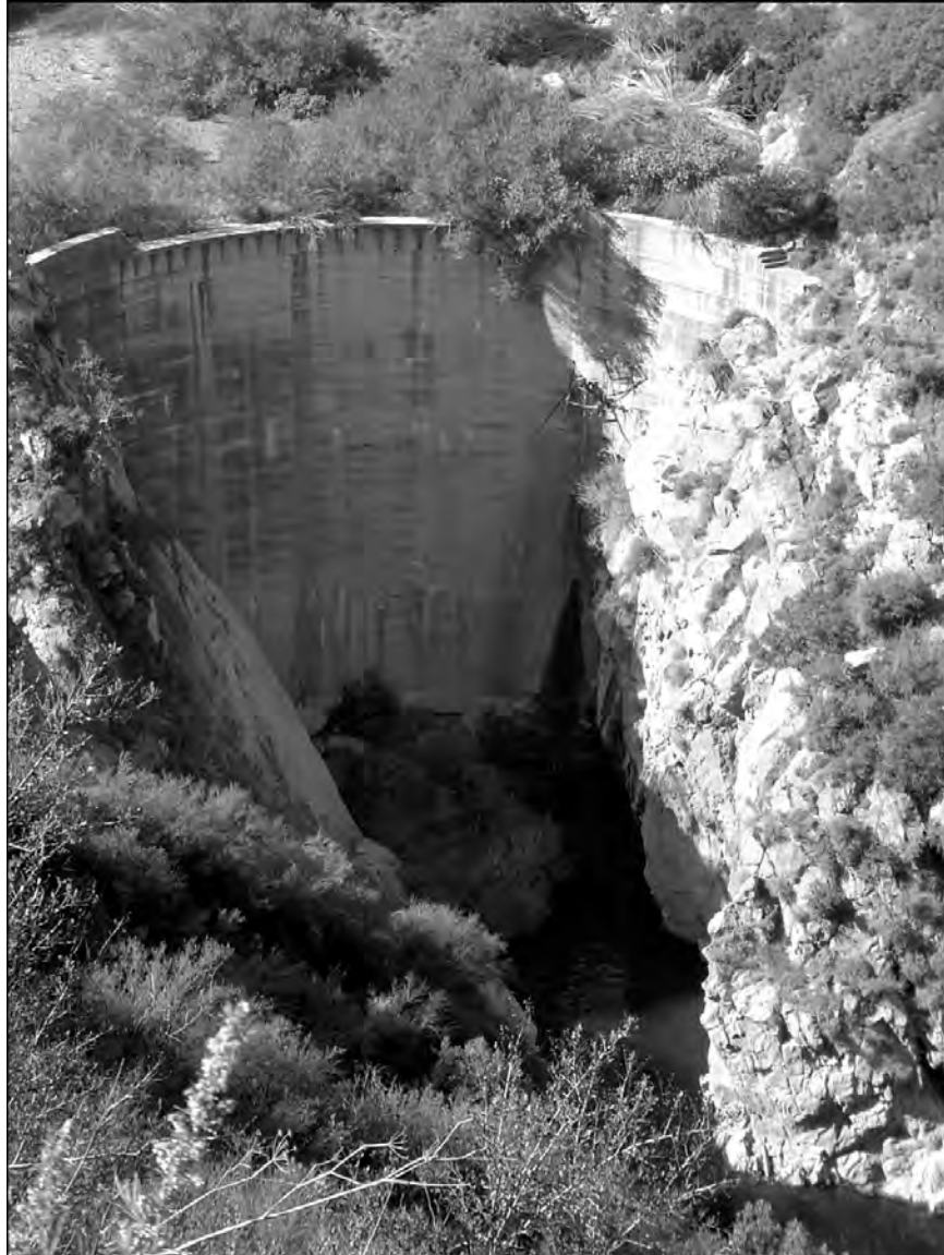
Figure 12. On the face of the dam, a portion of the water-distribution pipe and vertical-access structure remains.
