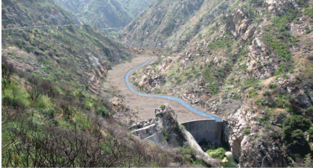
Figure 5.7-2 - Rindge Dam Mid-Point of Construction - 50% Removal
