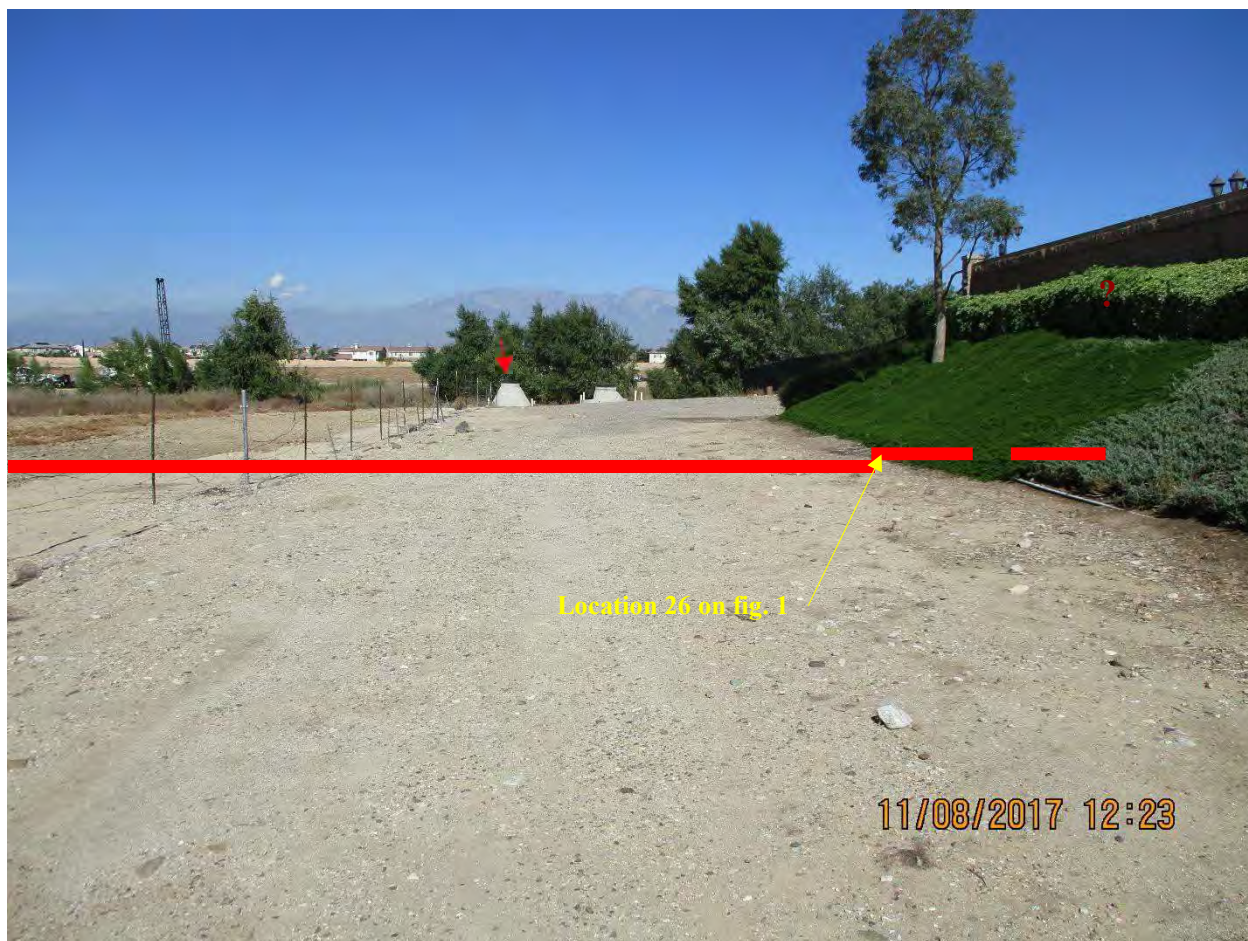
Fig. 33.—Looking due north at the southern abutment of River Road Dike conceptual alignments against the west face of a raised housing tract pad. Dike alignment represented by red line. Neither dike design width nor height determined as of the time of this writing. Note the sewer line manhole in the distance (red arrow) which represents a major sewer inceptor line; the dike crosses that sewer-line alignment approximately on perpendicular. 8 November 2017. Note the visible landscaping irrigation piping (white PVC) in the photograph at the bottom of the housing tract slope.
