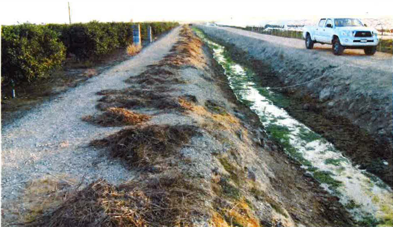
Photo 2: Typical cross section of Ferro Ditch facing downstream.
