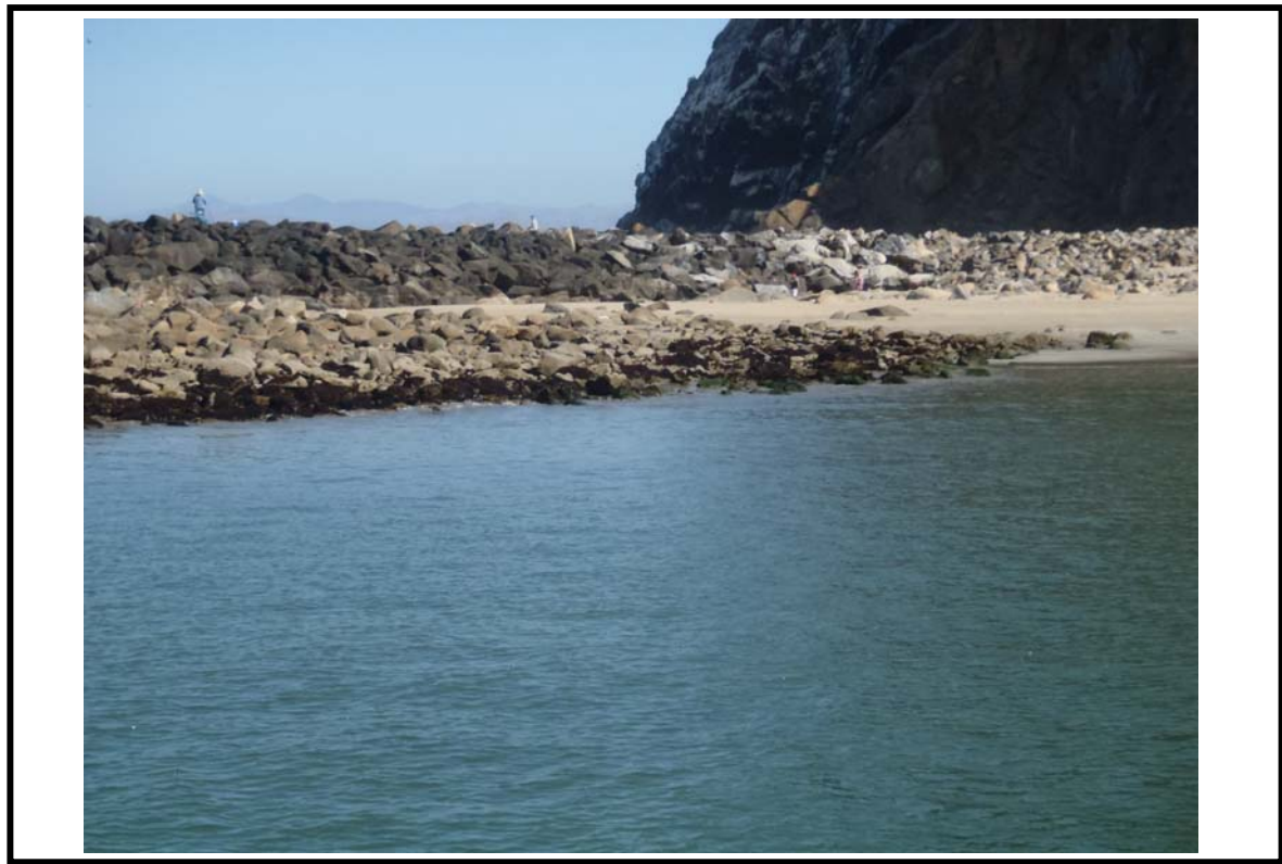
Photo 2b. Transition on north jetty from rip-rap to sand beach.
