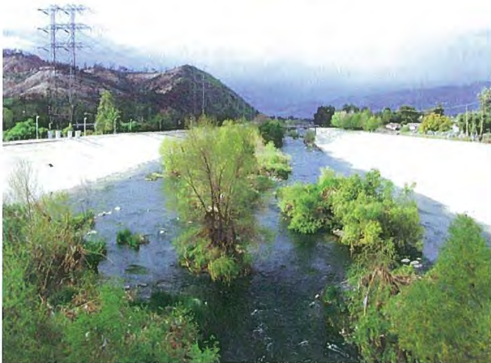
Figure 5. Examples of Fully and Partially Unlined Channel Reaches, Los Angeles River, California. Top: Sepulveda Basin, upper Los Angeles River (Approximate RM. 45.0) Photograph of the July 25-27, 2008 Los Angeles River Expedition. Bottom: Glendale Narrows (approximate RM 31.0).
