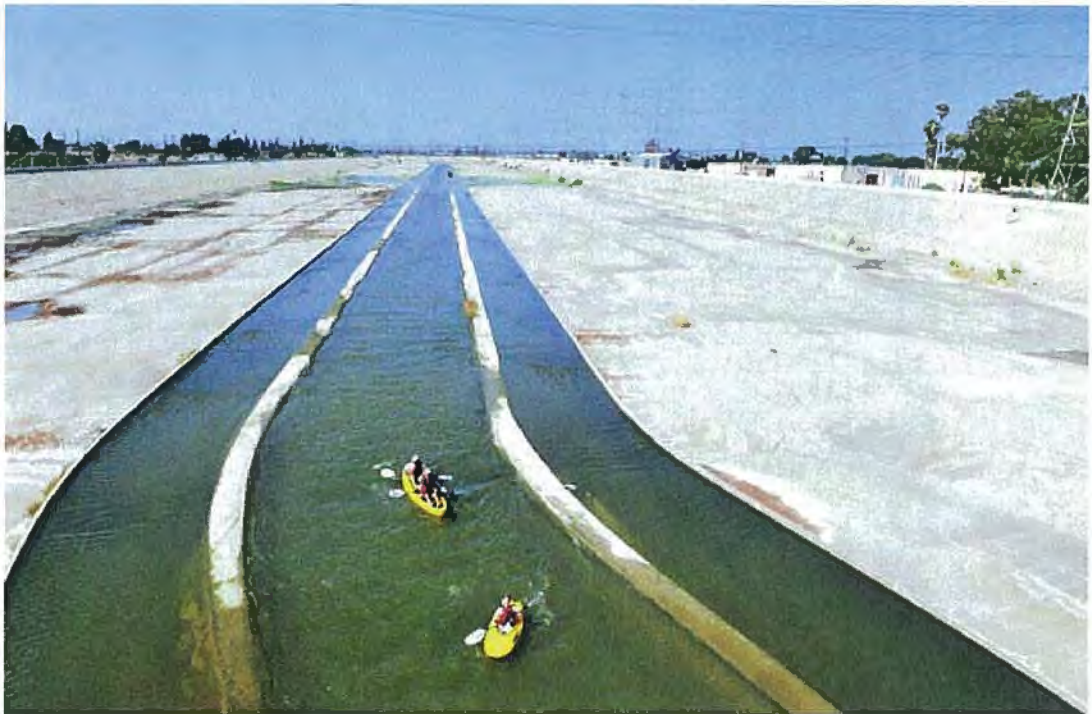
Figure 3. Photographs from July 25-27, 2008, taken by members of the Los Angeles River Expedition during the mid-point of the dry season. Examples of low flow channels embedded with larger concrete-lined flood channel. Top: Near the confluence of Arroyo Seeo at the Interstate 110 overcrossing (RM 24.7). Bottom: Typical 16-mile reach between Vernon and Long Beach (RM 3.2-19.2).
