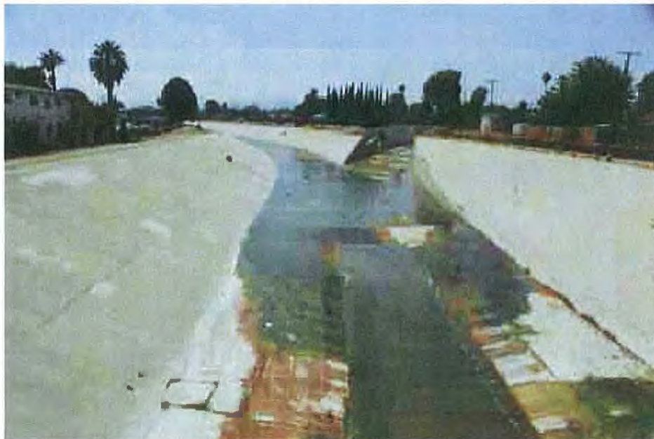
Figure 4. Top: Example of dry-season river reach with no low flow channel at the confluence of Arroyo Calabasas and Bell Creek at Owensmouth Avenue, the beginning of Los Angeles River (RM 51). Bottom: Looking upstream at transition between reach with no low flow channel and beginning of low flow channel at Mason Ave. confluence Canoga Park (RM 59.8).
